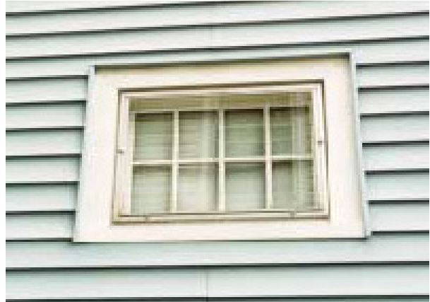
Exposed Window Frame
