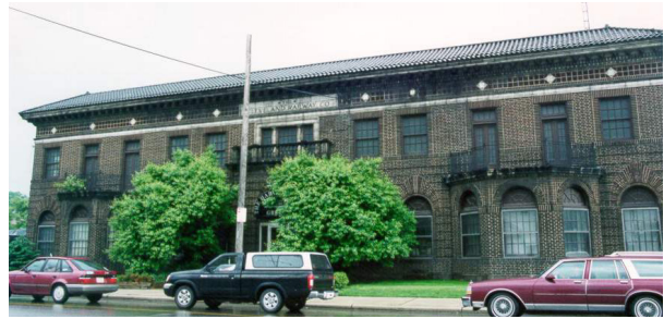
The Cleveland Railway Company Building, 5400 Harvard Avenue
