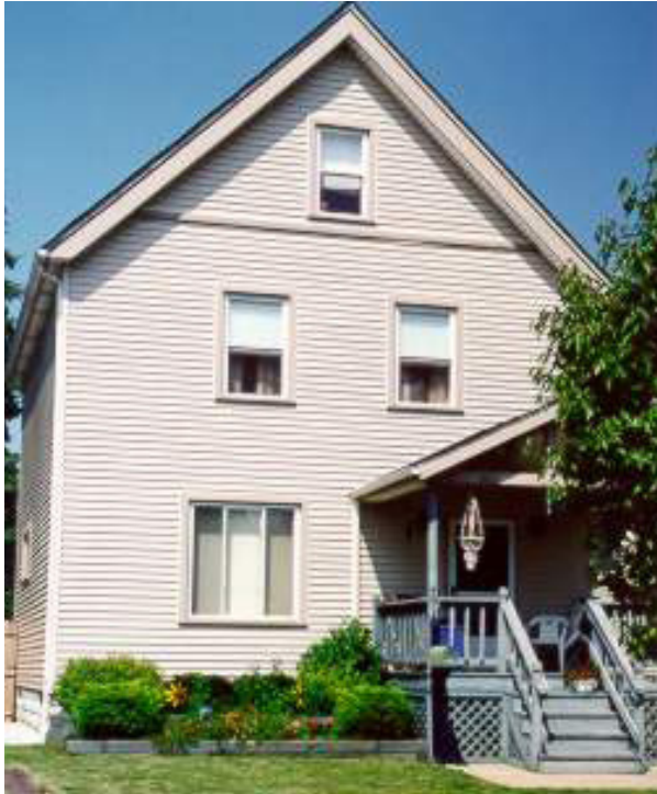
Inconsistent Window Sizes and Types
